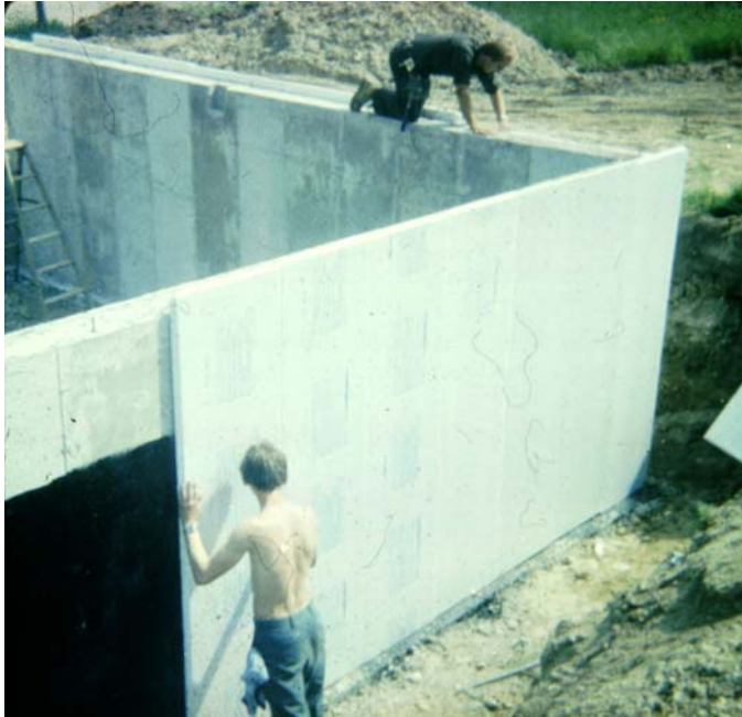
Photograph 1: Exterior Basement Insulation
