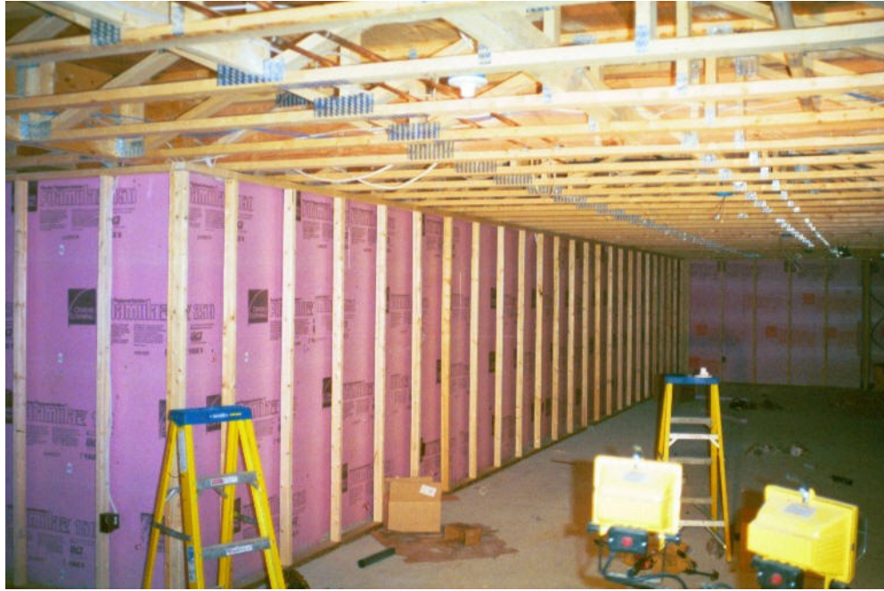
Photograph 4: Rigid Insulation/Frame Wall Under Construction
