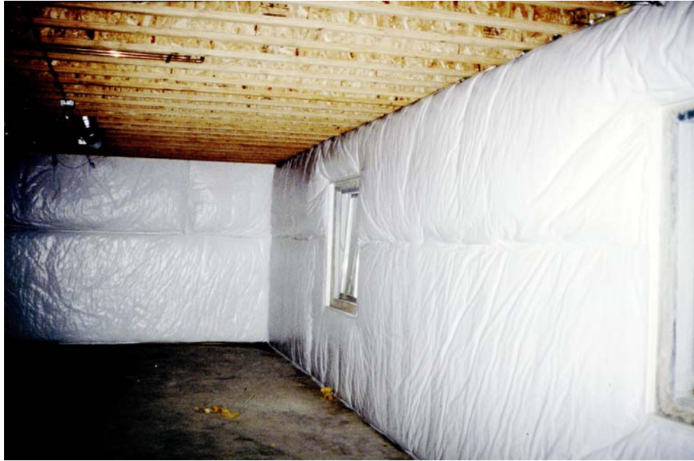
Photograph 3: "Blanket Insulation"
