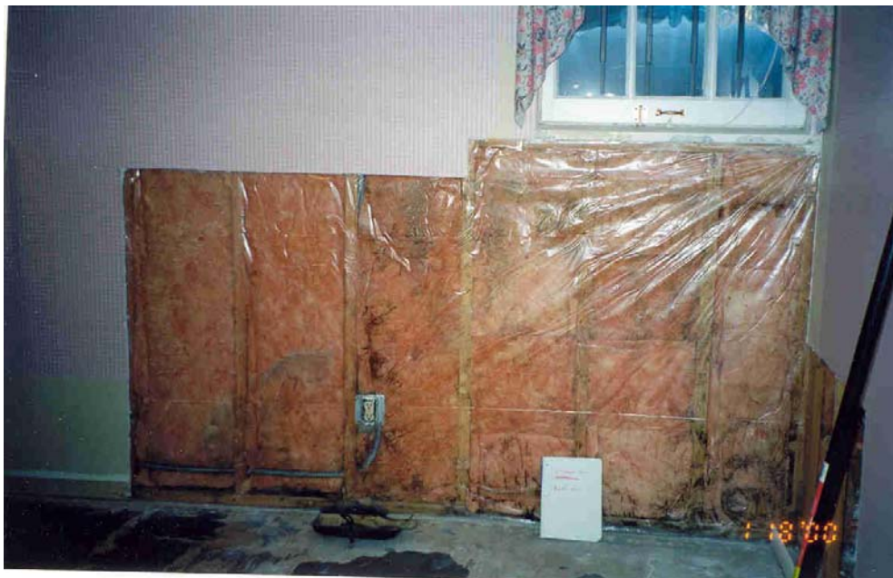
Photograph 2: Interior Frame Wall With Plastic Vapor Barrier
